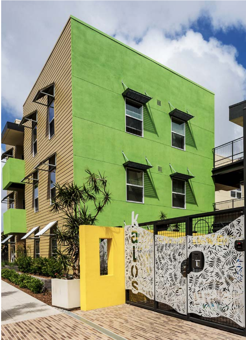
Kalos, a LEED Platinum Certified affordable housing community by M.W. Steele Group.
