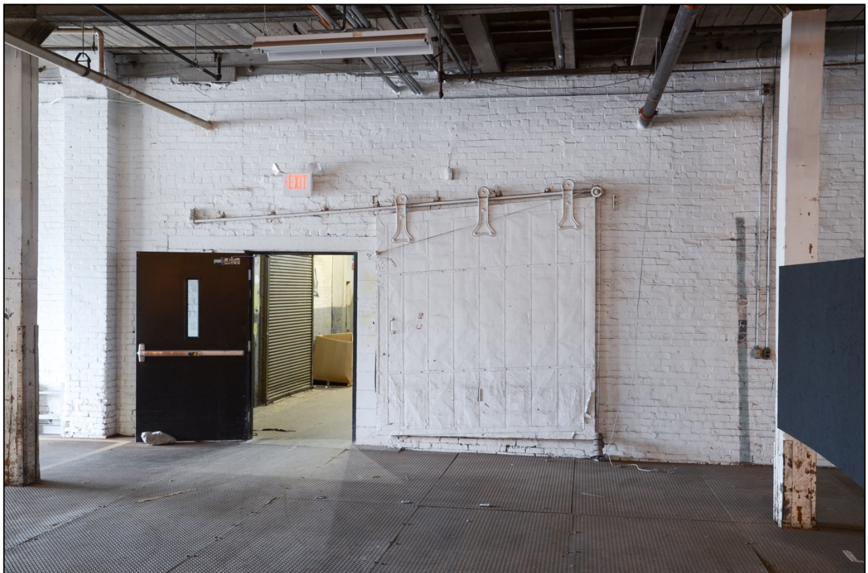
Figure 7. Sliding fire door, first floor, warehouse section.
