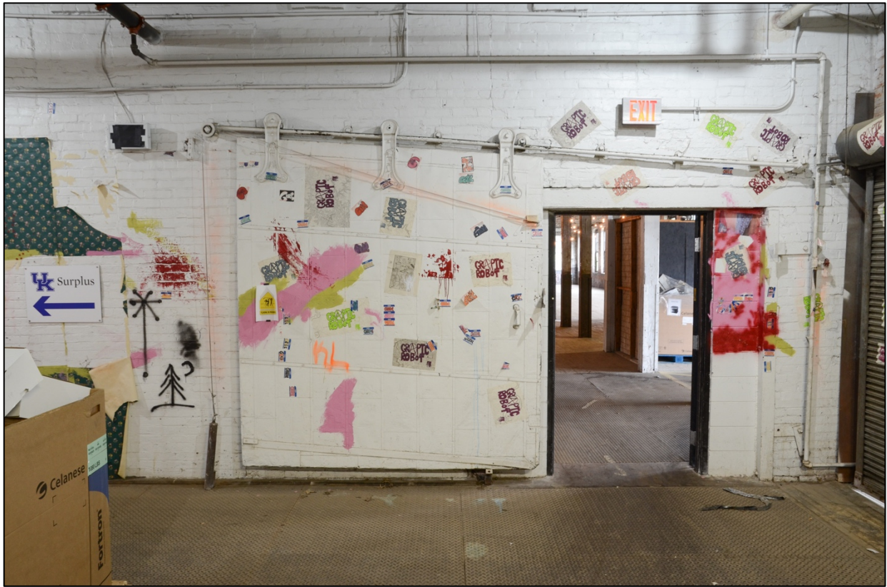
Figure 8. Sliding fire door, first floor.
