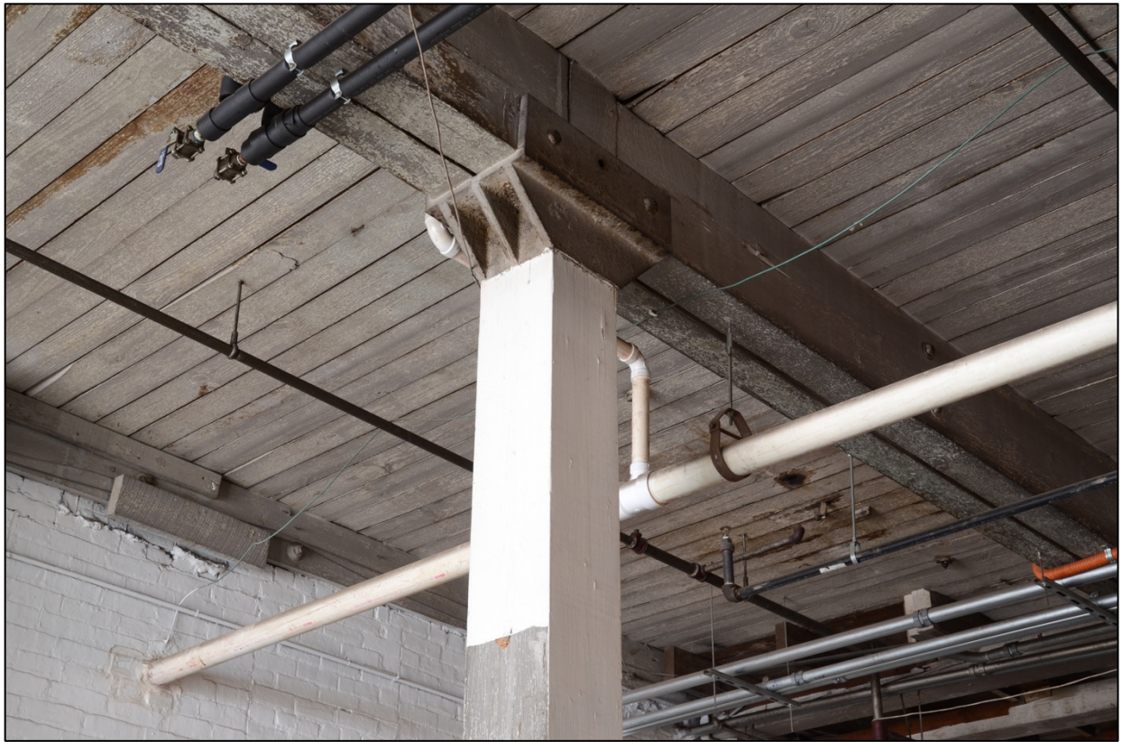
Figure 6. Heavy timber truss and bracket, warehouse section.
