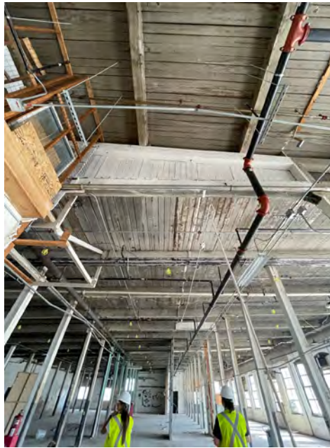
Water Damage & Chipping
